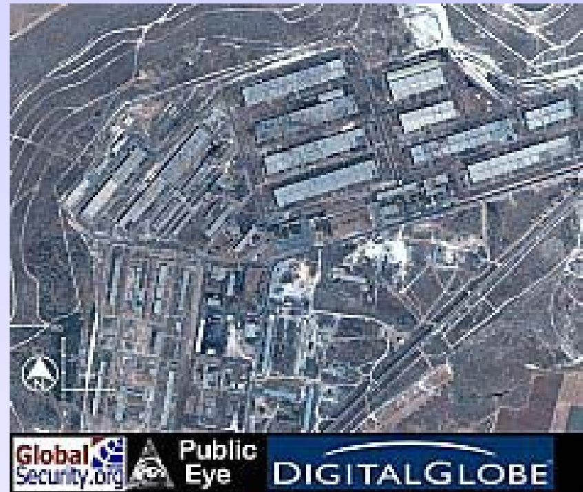
Al Safir CW plant
