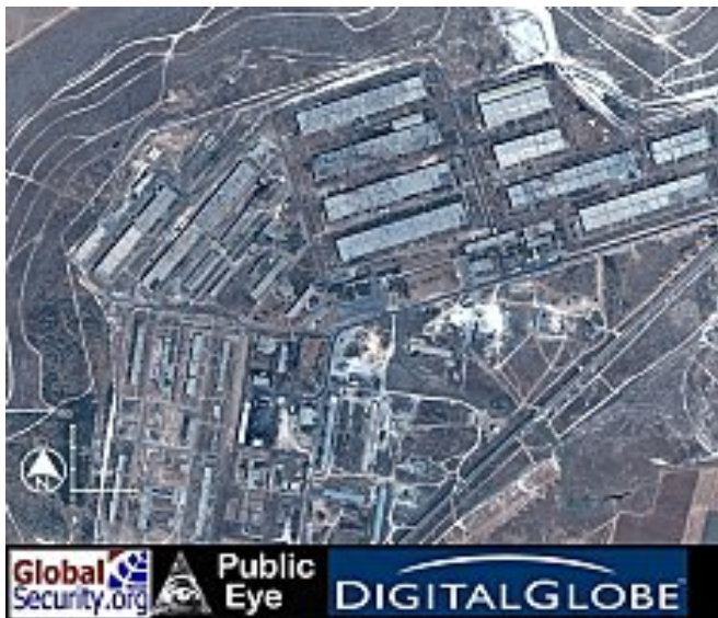
Al-Safir CW plant
