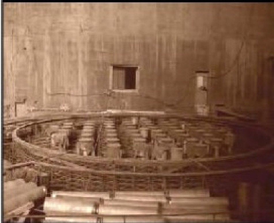
Top of the Syrian reactor before concrete poured.
